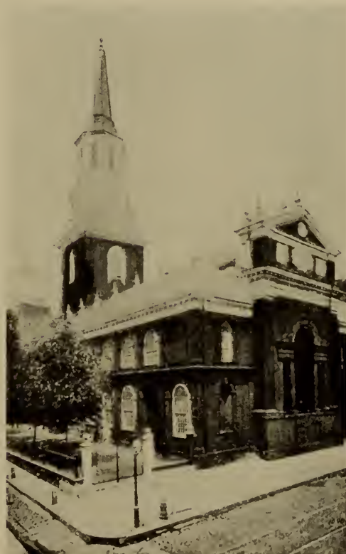
Christ Church, now tucked away in the incongruous, uncongenial mercantile district of Philadelphia.
